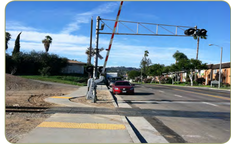
Figure 4.9: The Idaho Street railroad crossing
