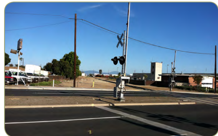
Figure 4.16: Looking east from Harbor Boulevard railroad crossing
