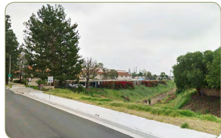
Figure 6.2: The Carbon Creek Channel ROW from Imperial Highway
