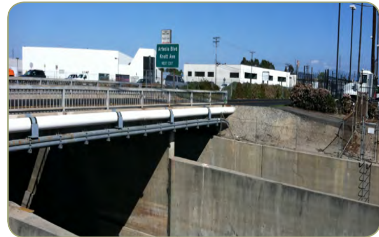
Figure 3.14: The Firestone Boulevard South Overpass
