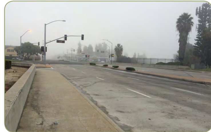
Figure 3.34: Looking east along Alondra Boulevard towards the Stage Road intersection
