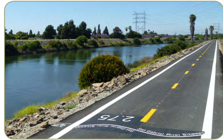
Figure 1.13: San Gabriel River Bikeway, scenic area which may not require landscaping (image from Wikipedia)
