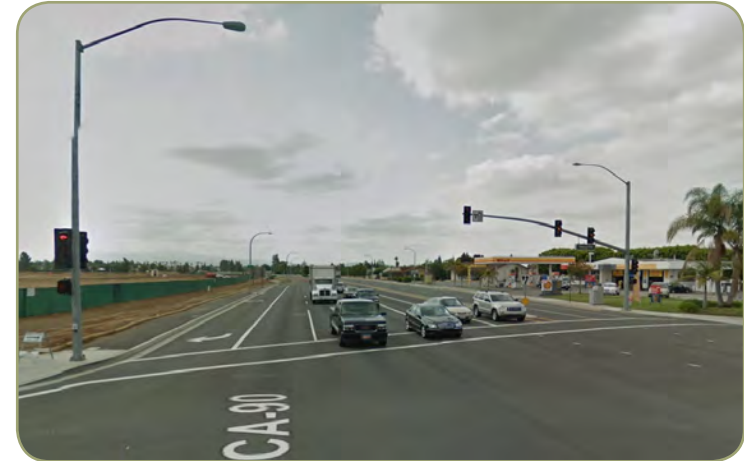
Figure 6.1: Imperial Highway from Valencia Avenue with the La Floresta development construction visible on the left
