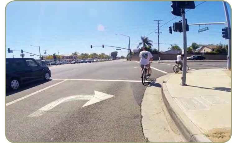
Figure 8.11: Pacific Coast Highway at Seal Beach Boulevard. Note the right turn lane displacing the bike lane.
