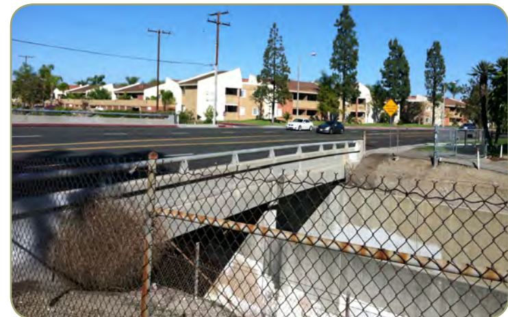
Figure 3.24: Stage Road overpass
