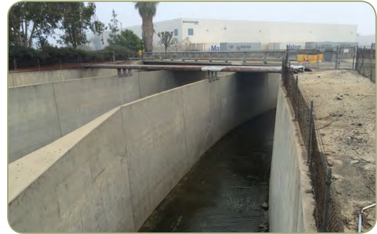
Figure 3.16: The Trojan Way Overpass as seen from the Firestone Boulevard overpass
