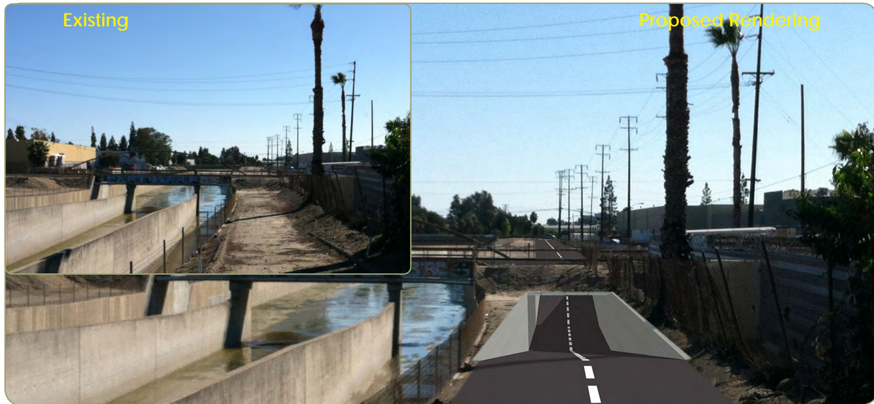
Figure 3.20: Looking south from Firestone Boulevard South with existing conditions (top left) and proposed OC Loop, excluding wayfinding and landscaping
