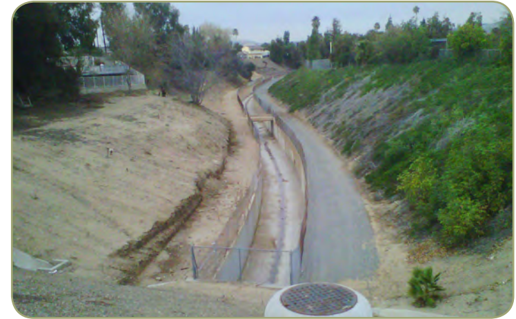
Figure 6.4: Looking north along the Carbon Creek Channel ROW from Bastanchury Road
