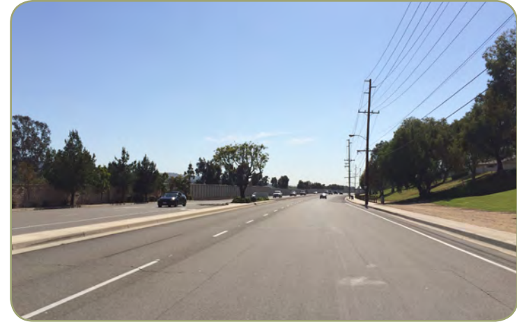
Figure 7.18: Looking west on Esperanza Road from the Fairmont Connector with bike lane and El Cajon Trail facilities visible
