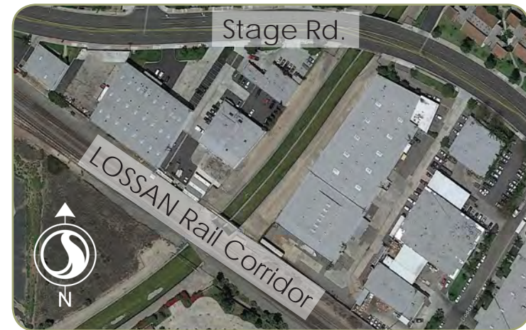
Figure 3.23: LOSSAN Rail Corridor Crossing to Stage Road
