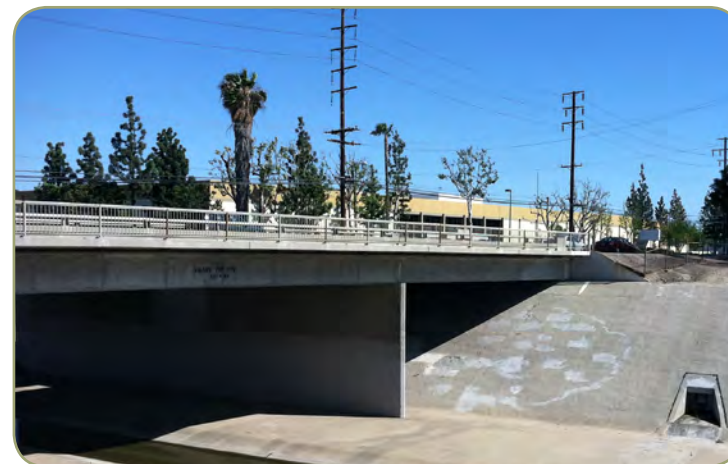
Figure 3.6: The Valley View Avenue Overpass
