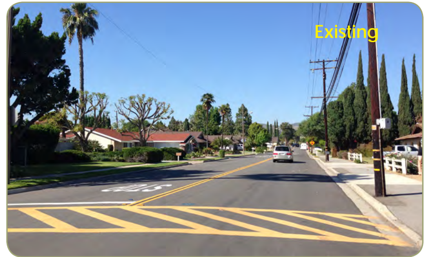
Figure 7.12: Grandview Avenue existing conditions looking eastbound
