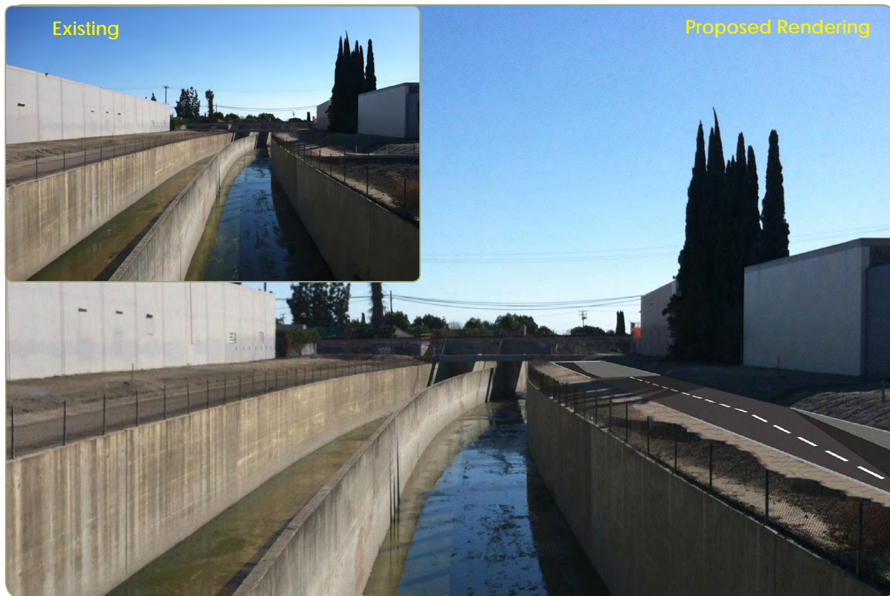
Figure 3.32: Looking south towards the LOSSAN Rail Corridor from Stage Road with existing conditions (top left) and proposed OC Loop Bikeway excluding wayfinding and landscaping
