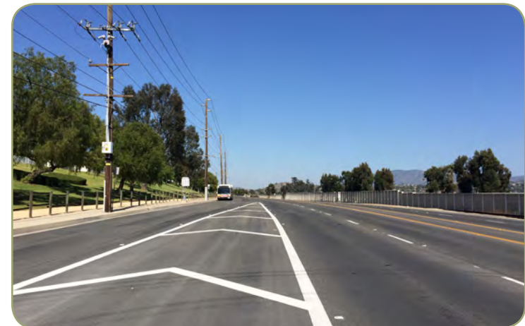
Figure 7.16: Looking eastward along Esperanza Road from Fairlynn Boulevard with buffered right turn lane and existing Recreation Trail visible on the left
