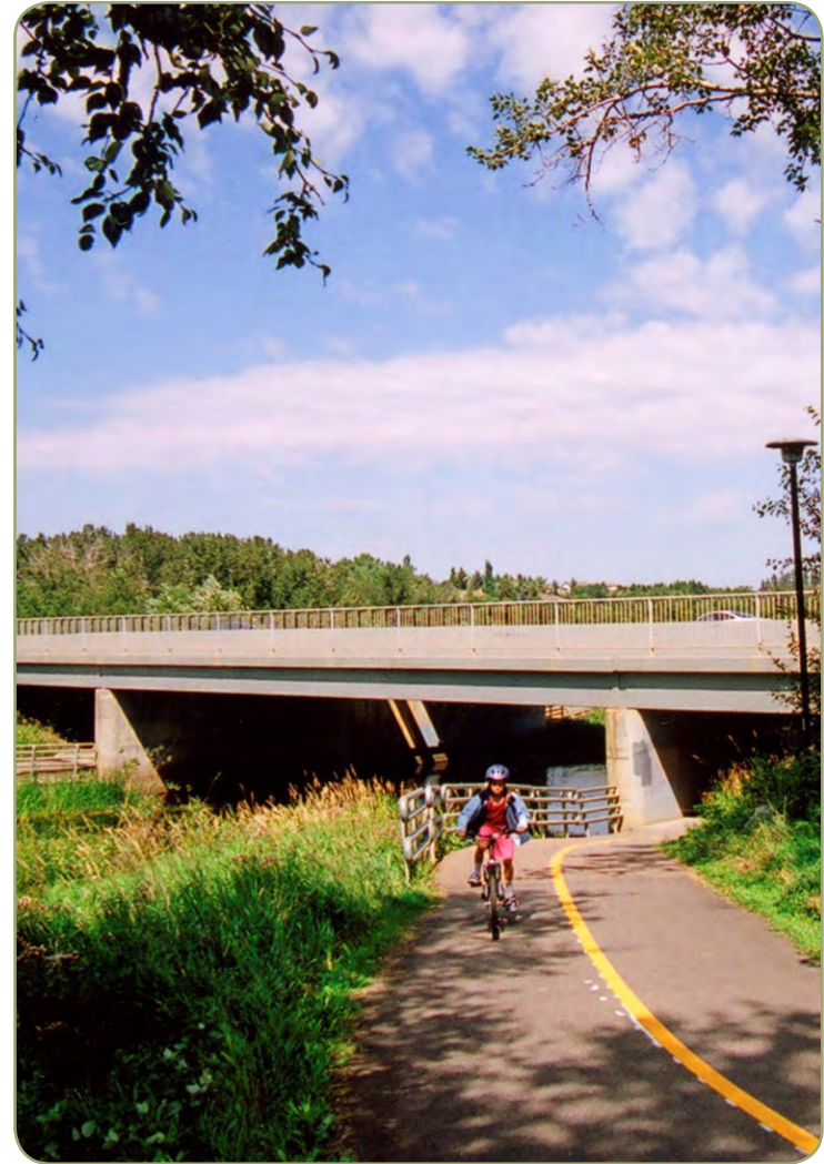
Figure 1.10: Sample class I bicycle underpass (from Bousdreau Bridge in St. Albert, Canada)
