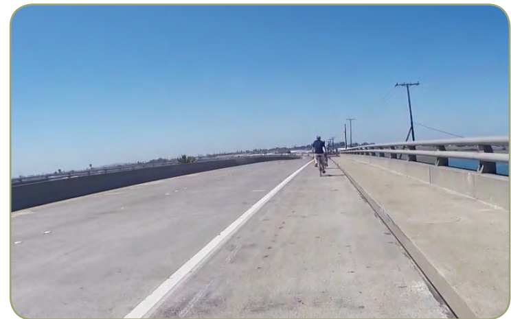
Figure 8.10: The Pacific Coast Highway Bridge over Anaheim Bay
