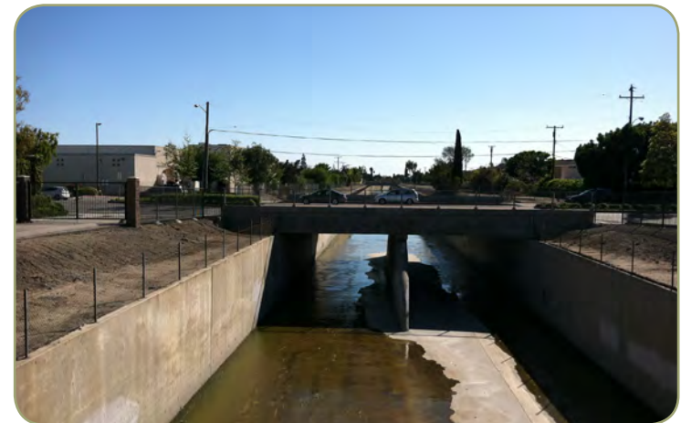
Figure 3.26: The La Mirada Boulevard Overpass
