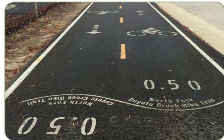
Figure 2.7: Existing bikeway branding and mile marker wayfinding elements along the North Fork Coyote Creek Bike Trail
