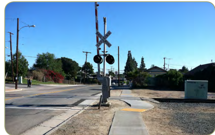
Figure 4.12: Looking south from the Walnut Street railroad crossing
