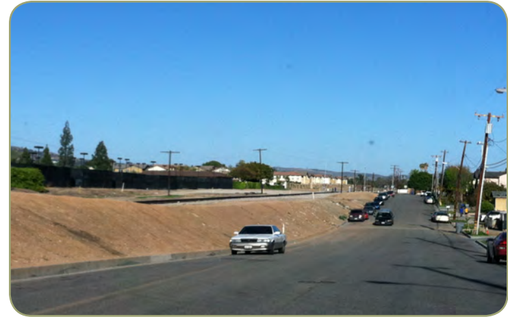
Figure 4.13: Looking east down Electric Avenue
