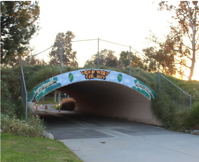
Mile Square Regional Park - Pedestrian Bridge, 2019
