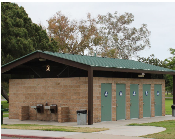
Mile Square Regional Park - Restroom Structure, 2019
