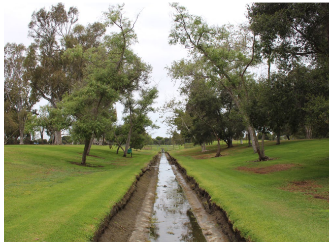
Mile Square Regional Park - South Storm Drain, 2019
