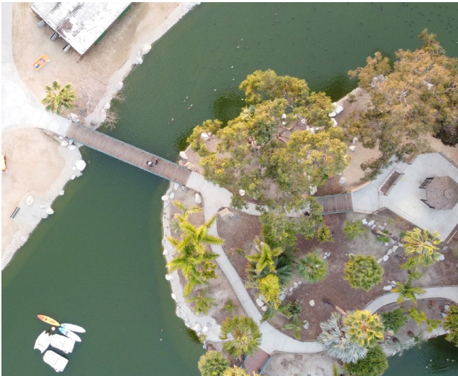
Mile Square Golf Course - North Pond Bridge, 2021
