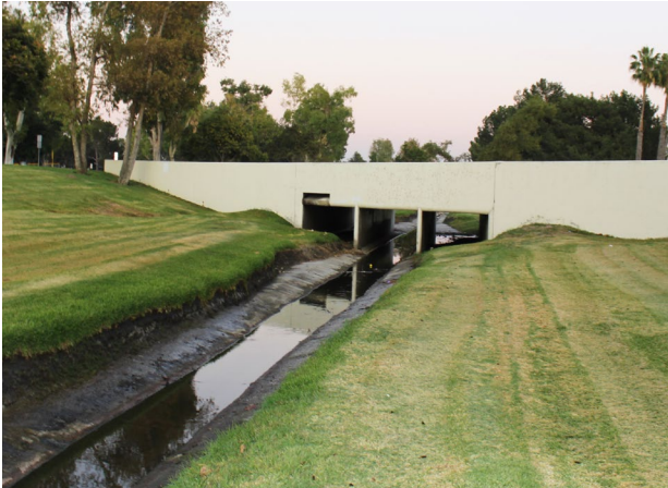
Existing Drainage Channel and Circulation Bridge
