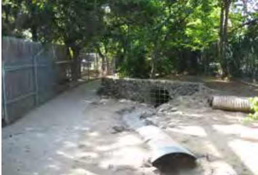
B Drainage Outlet
