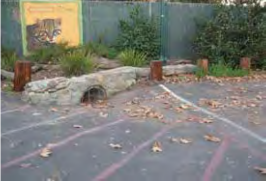
A Drainage Inlet
