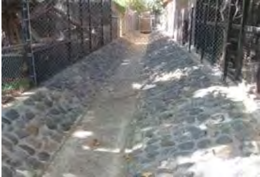
Concrete/Grouted Rock Drainage Swale (spans A-B)
