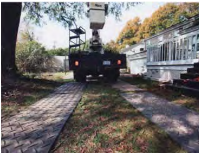
AlturnaMATS prevent damage to root zones around trees.
