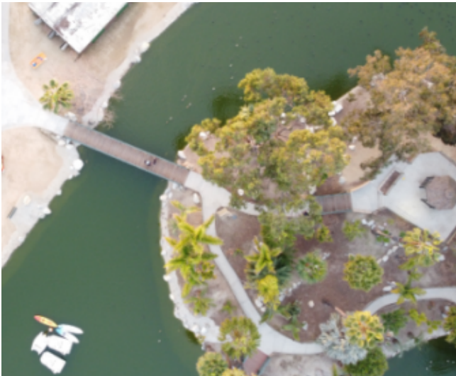
Mile Square Golf Course - North Pond Bridge, 2021
