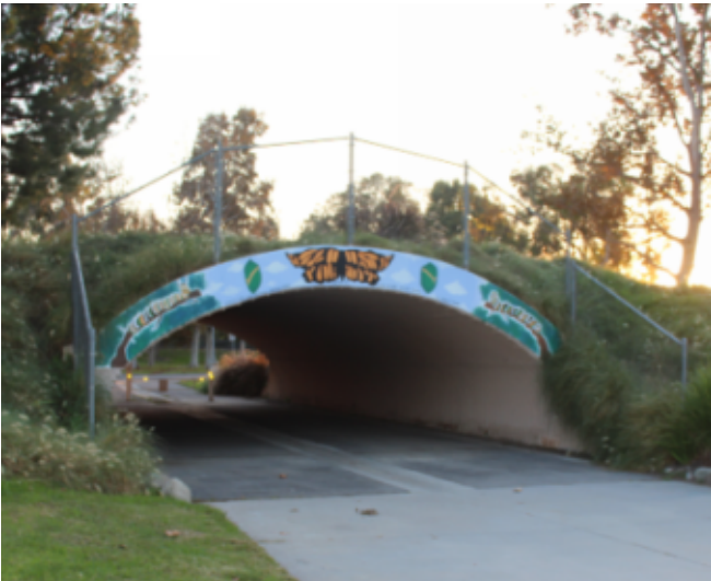
Mile Square Regional Park - Pedestrian Bridge, 2019
