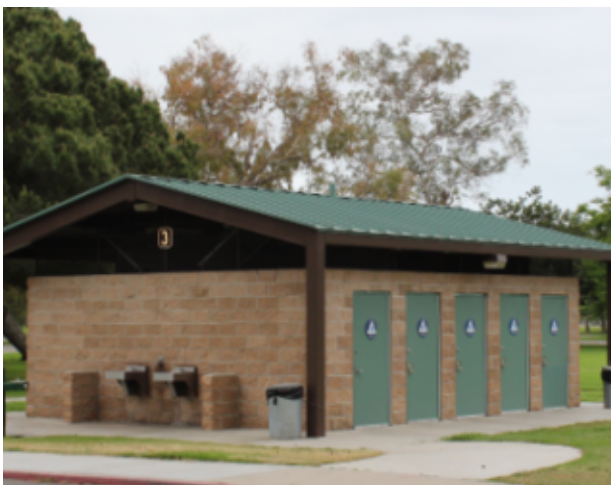
Mile Square Regional Park - Restroom Structure, 2019
