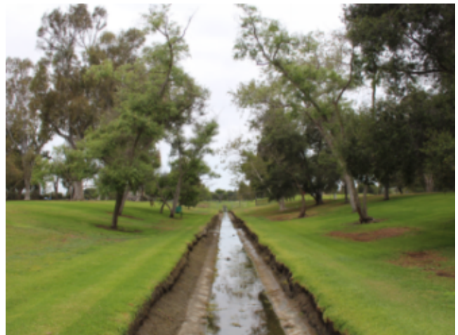
Mile Square Regional Park - South Storm Drain, 2019
