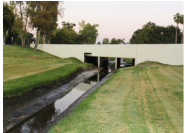
Existing Drainage Channel and Circulation Bridge
